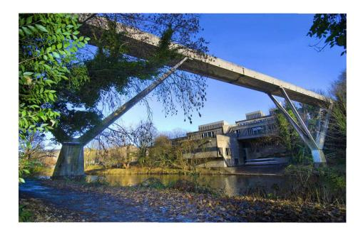
Kingsgate Footbridge in Durham is a grade 1 listed reinforced concrete bridge structure built in 1963. The bridge spans the river Wear and links the University and Durham Old Town.
