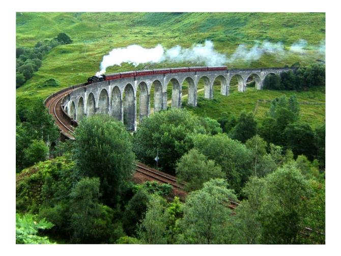
The Glenfinnan Viaduct stretches 416 yards along an elegant curve rising 100 feet above the head of the River Finnan Valley in Inverness-shire. It was built in the late 1890s as part of the West Highland Railway (the "Iron road to the Isles"). One of a number of structures built along this section of the line, it stands above the Glenfinnan Valley at the head of Loch Shiel, close to where Bonnie Prince Charlie raised his standard of rebellion in 1745.
