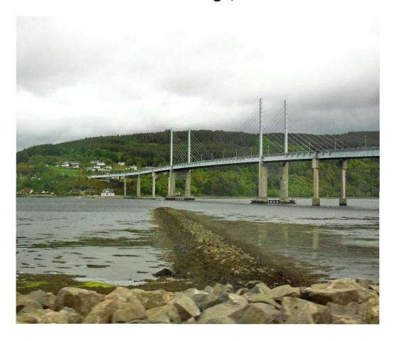
The Kessock Bridge carries the A9 trunk road over the Beauly Firth between Inverness and the Black Isle replacing the former ferry. When built from 1978–82 it was the largest cable-stayed bridge in Europe and the only one of its type in Britain. Its design is said to have been modelled on the Rees Bridge over the Rhine near Dusseldorf.
